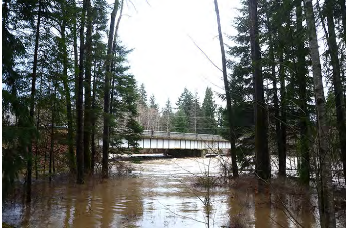
Figure 2: High Water on Oyster River at Highway 19 Bridge, December 2014 (Campbell River Mirror, 2014)
